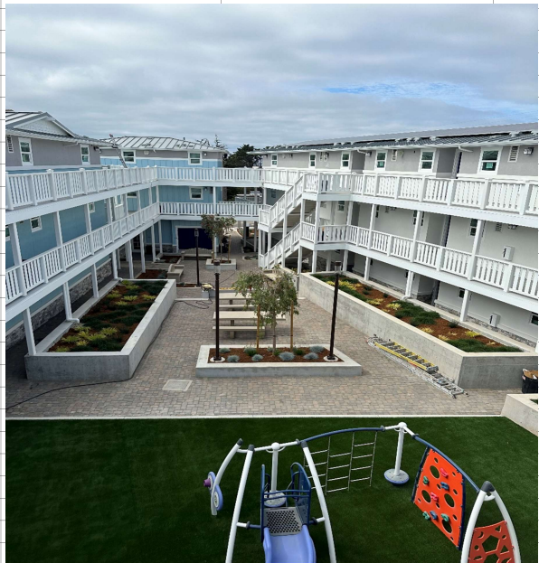
Morro with turf installed
