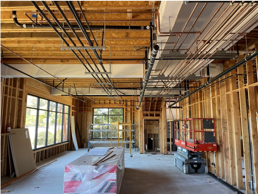
Ironworks Mixed Use
