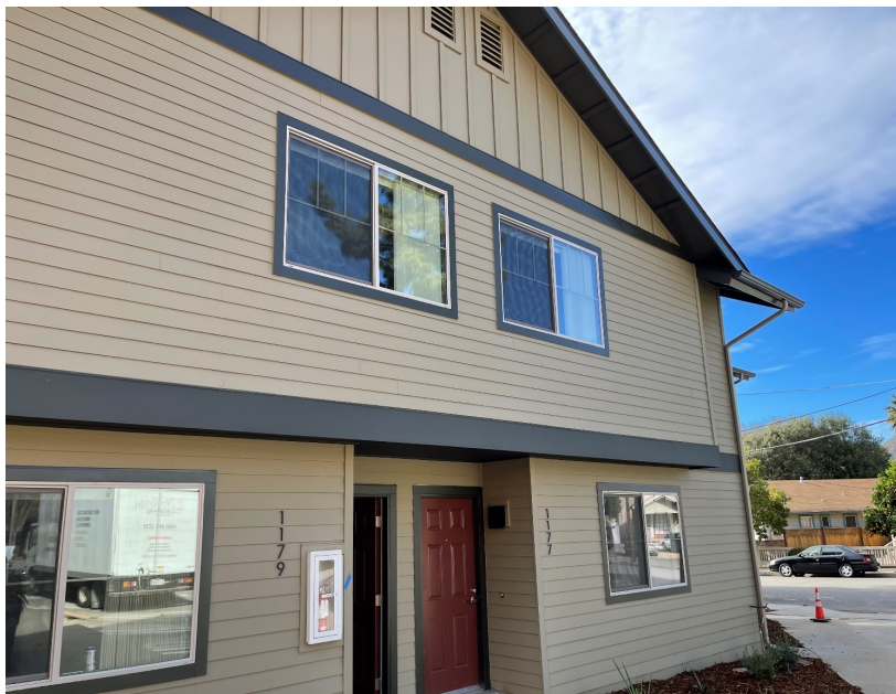
Arbor Place Exterior Renovation
