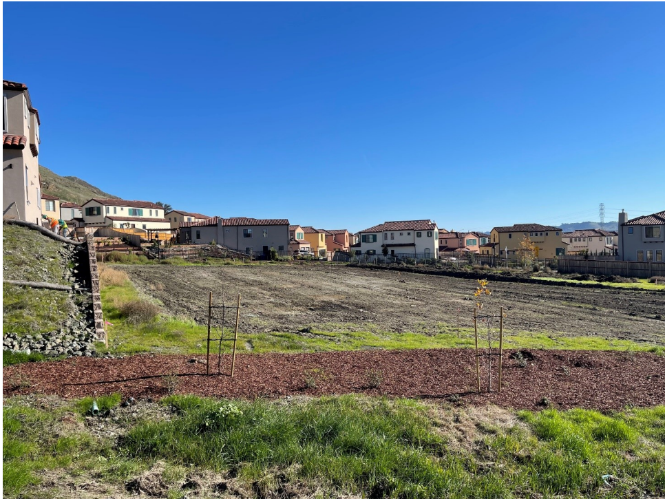
The Apartments at Toscano
