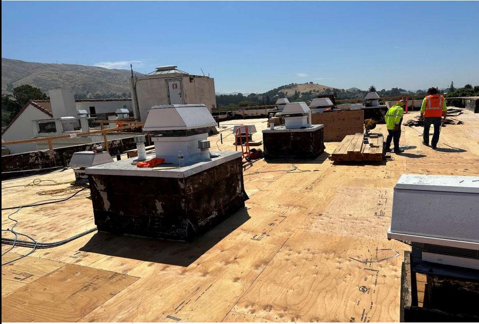
Anderson - new roof sheathing
